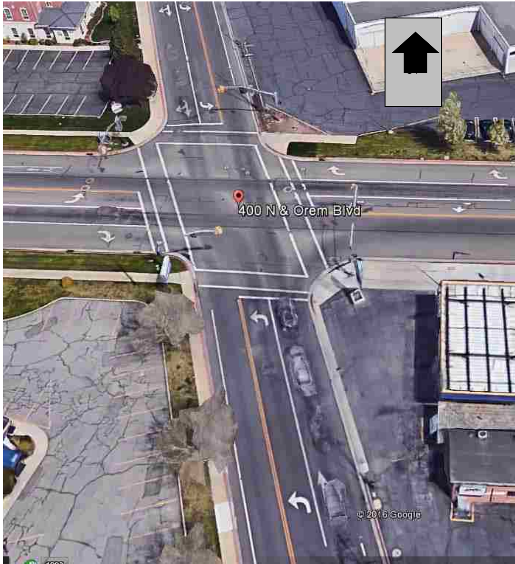
Figure 2-6: Example of a left-turn bay in Orem, Utah (Google Earth 2016).
